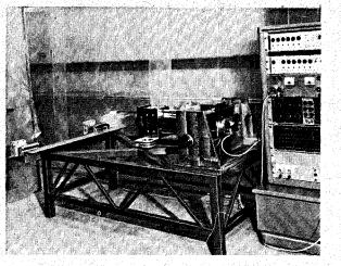
Fig. 9. Automatic position control system using trilateral co-ordinates.
