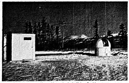
Fig. 10. The Whitehorse satellite tracking station in the Yukon. Precision cameras photograph the relative positions of the satellite and its star background.
